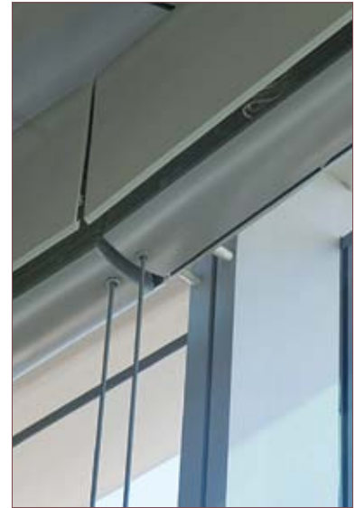
Custom pelmet/fascia on a curved facade.
