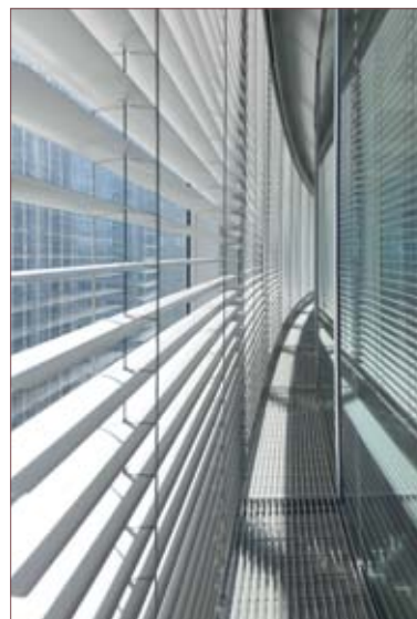
The ladder braid attached to omega punch ensures correct spacing between slats.
