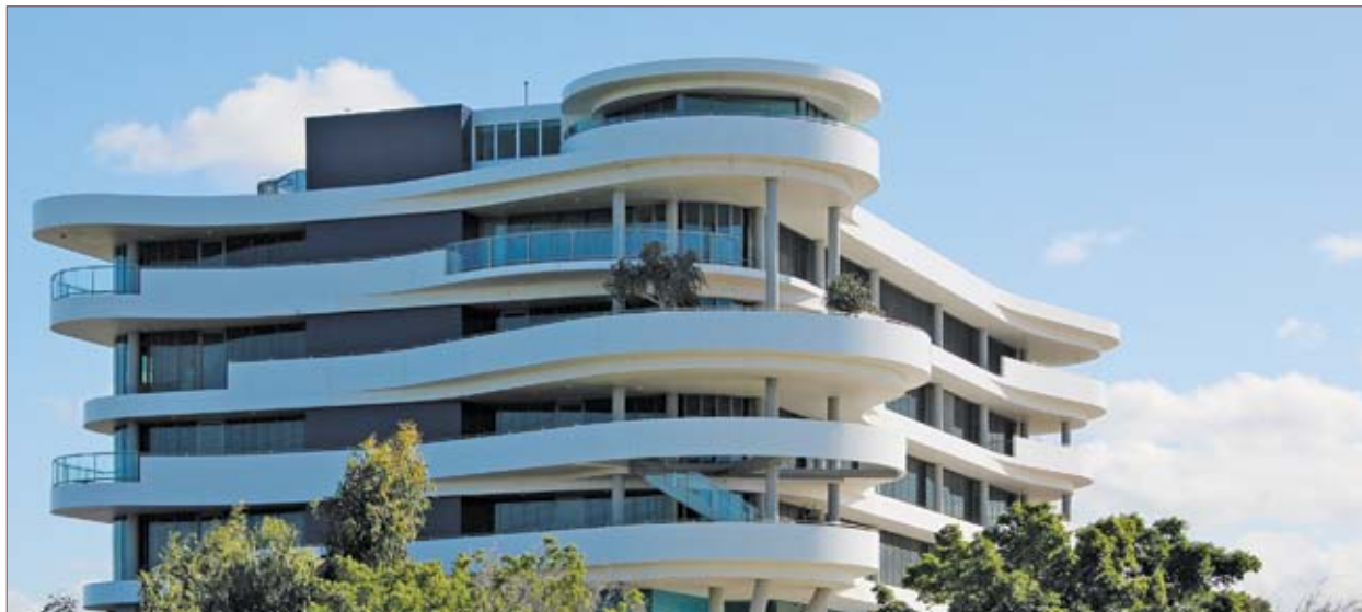
Retractable Horizontal Louvers - external. Port authority building in tropical environment.
