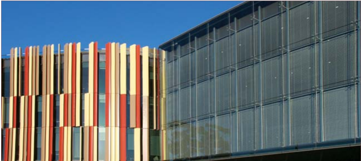
Retractable Horizontal Louvers - internal. University building.
